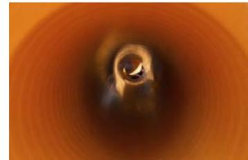
Inflatable packers are used to allow flows to continue to pass through the system whilst the patch liner has been inserted in the defective areas allowing the continued use of the system. This reduces the impact on customers, allowing continued use of their internal facilities.
